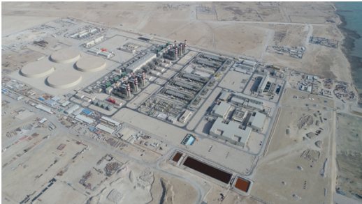
Umm Al Houl Power, Qatar
